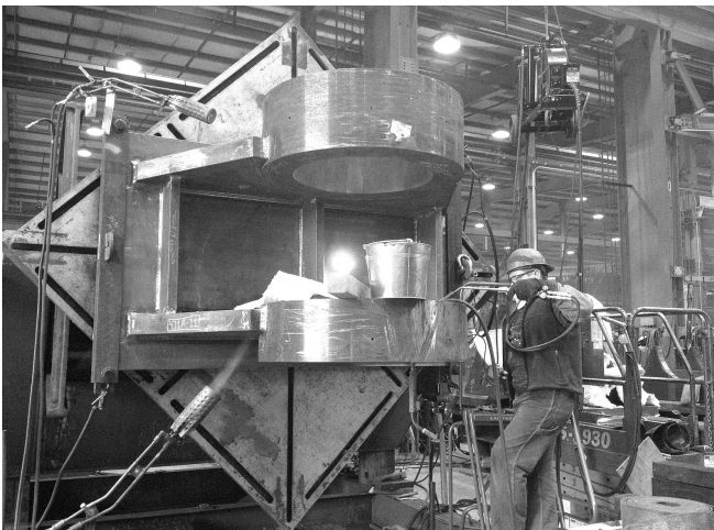
A crew member welds together metal on the pin pedestal for the new Folsom Dam auxiliary spillway Nov. 28, 2012, at the Oregon Iron Works' Clackamas. Credit U.S. Army Corps of Engineers Sacramento District
